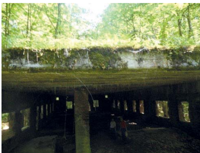
Fig. 9. View of the slab with pre-tensioned beams and concrete topping
